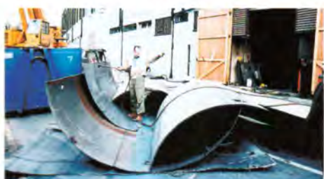
Demolition of the boilers
