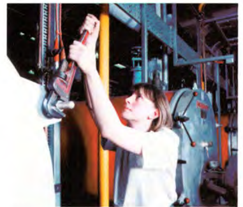
1992. RAE CALCUTT, adjusting boilers in King Edward Building.
