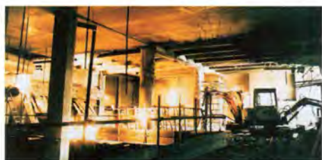
Removing the chimney stack
